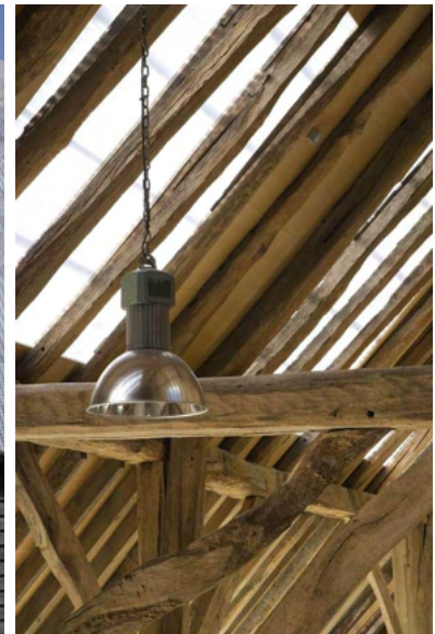
Figure 14. The interior of the same barn from Fig. 13. Note that harsh, direct sunlight is made soft and indirect with the small perforations of the panels.
