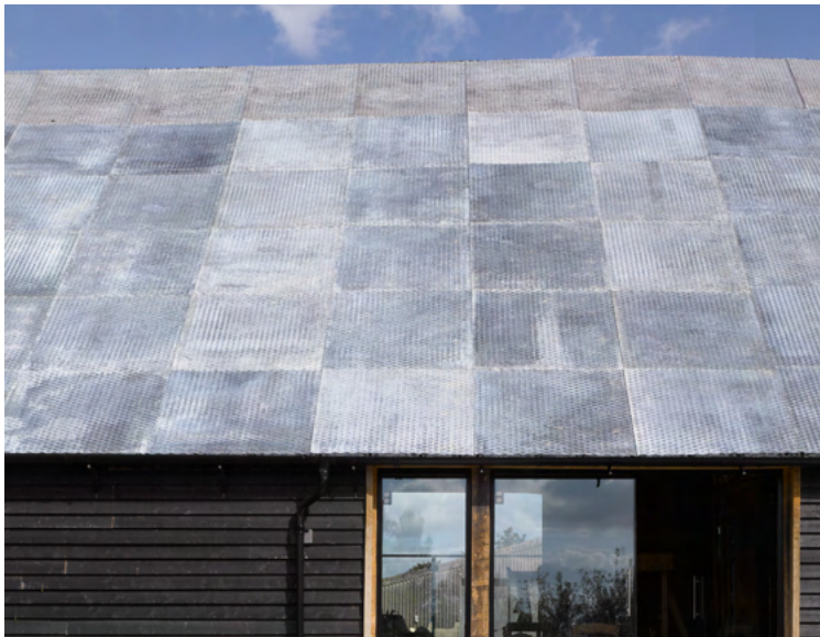
Figure 13. Perforated aluminum roofing panels allow lighting to pass through to the interior without compromising the historic character of this restored barn.
