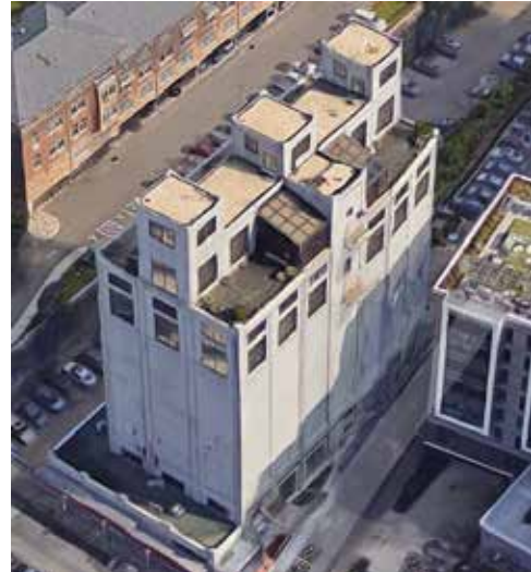
Reading Company Grain Elevator. Courtesy Google Earth Streetview.
