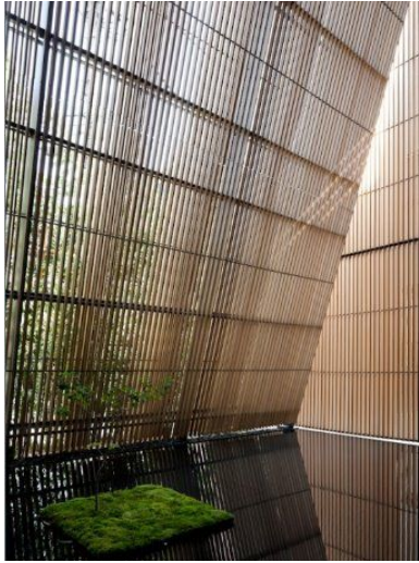
Figure 11. Natural lighting softened by wood screens in the Hiroshige Museum, Japan.
